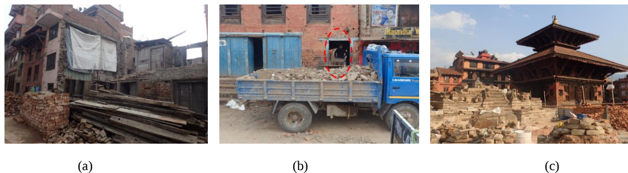
Figure 3: (a) Damaged buildings and materials in Khokana, (b) debris removal from a house in Bhaktapur, and (c) damaged monument reconstruction in Bhaktapur
