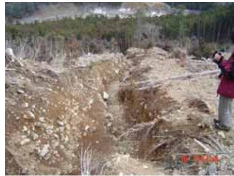
Photo 4 A gully on the slope near Miyagawa Reservoir
