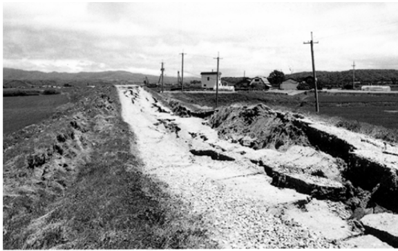
Figure 9 Damage to a dike at the Shiribeshi-toshibetsu river, Hokkaido, Japan, during 1993 Hokkaido-Nansei-oki earthquake
