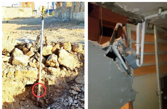
Fig. 1.8. Damage to joint of the gas pipeline at the entrance to the houses at Sarpole-Zahab city.
