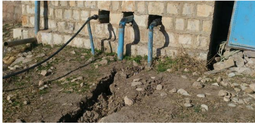
Fig. 1.7. Damage to the Gurchi-Bashi village vessel and Pipeline due to settlement and landslide in some parts.
