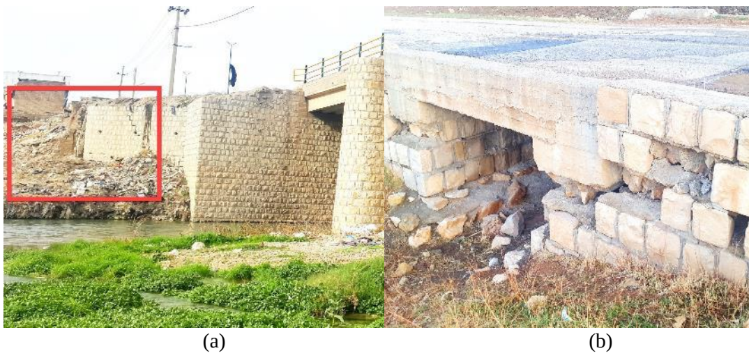
Fig. 1.2. (a) Damage to the retaining walls beside the bridge of Sarpole-Zahab City, (b) damage to little stone and concrete bridge at a Village road nearby Sarpole-Zahab [13].
