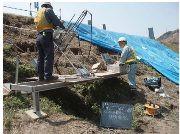
Fig. 4 Inclination measurement by NSWS testing machine
