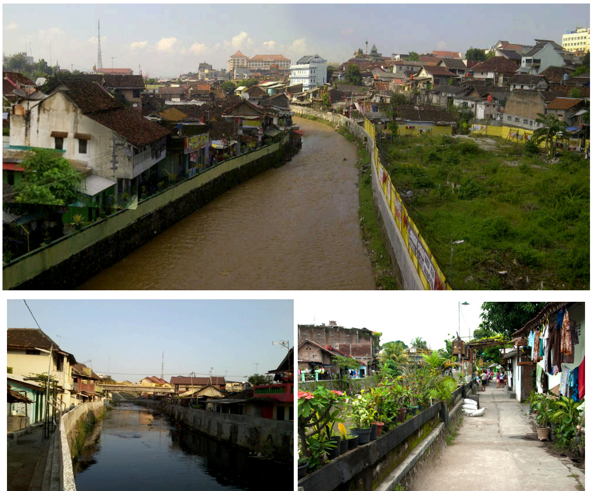
Figure 3-4 Existing condition of riverside area in Yogyakarta City
