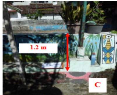
Figure 2-14 Heightened floodwall (Sukoco, 2013)
