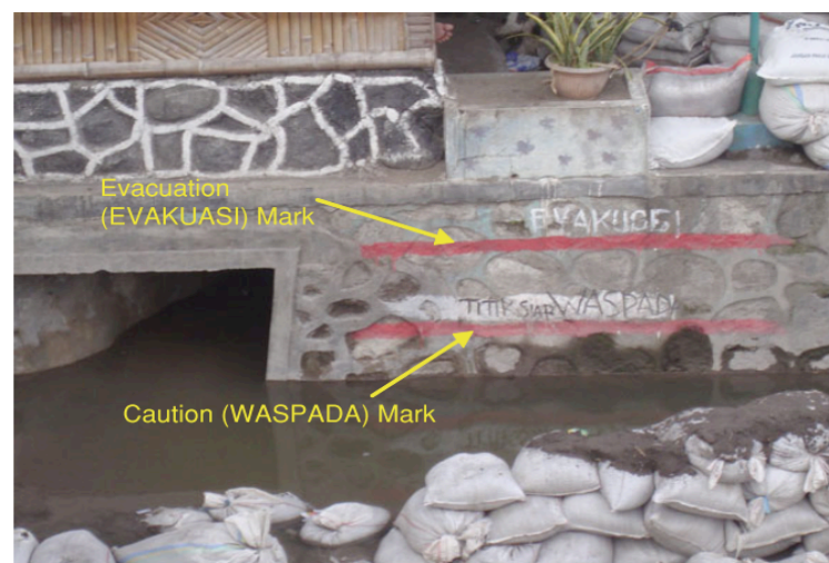
Figure 2-12 Water level mark on the levee as monitoring and early warning (Fathani and Legono, 2012)
