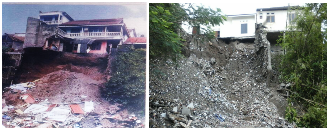
Figure 2-11 Landslide event in Code River
