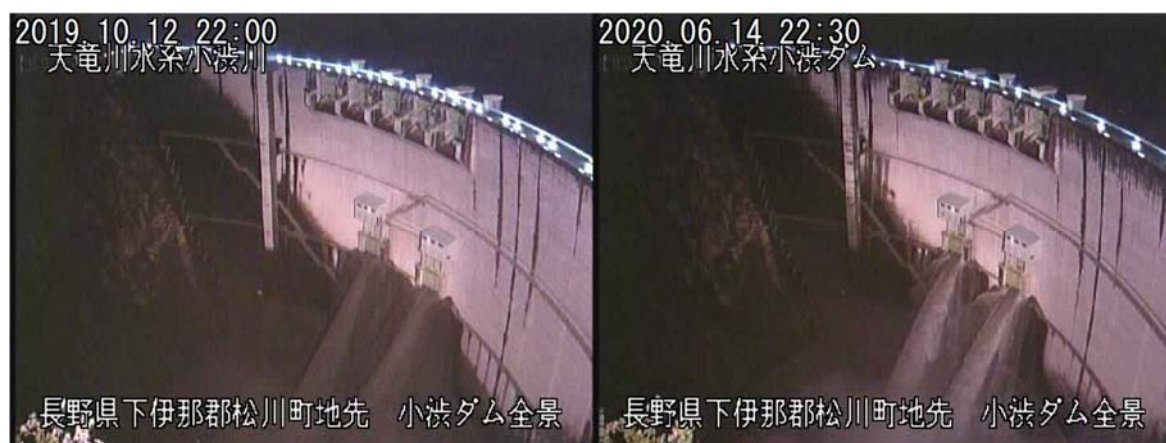
Fig. 8 Flow release from conduit gates of Koshibu during the typhoon (left) and different flood (right).
