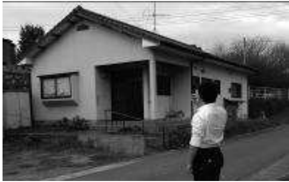
Photo 1 Collection of house façade
