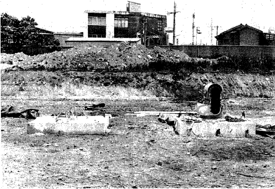
Photo. 2 Active (F2) and passive (F3) foundations
