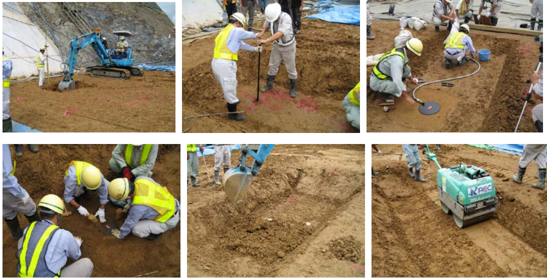
Figure 3.20 Procedure for installing WPT with earth pressure transducer
