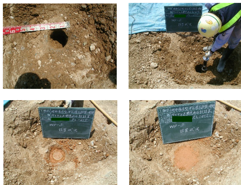
Figure 3.12 Outline of WPT installation in core zone
