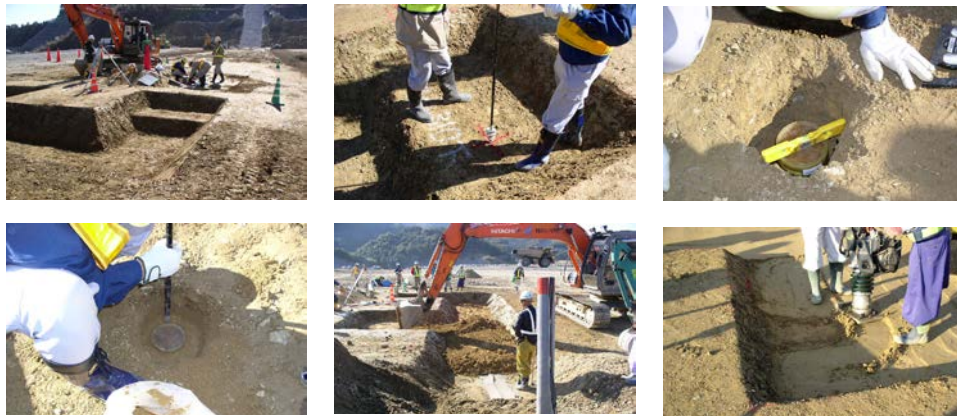
Figure 3.6 Procedure for installing WPT (core boring method)
