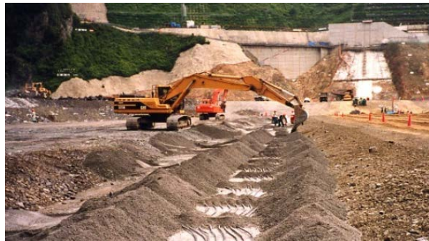
Figure 3.1 Cable trench for installing sensors
