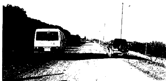
Photo 1 Jingjiang great dyke
