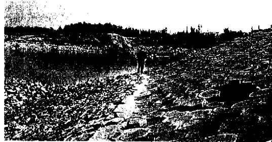
Photo 7 Protected bank erosion (Shishou)
