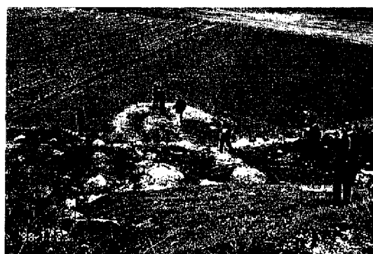
Photo 5 Sediment deposition due to piping at the base of a dyke (Yueyang)
