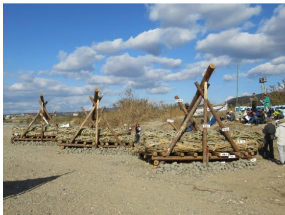
Photo 6 Seigy (crib spur) set up in the Kizu River
