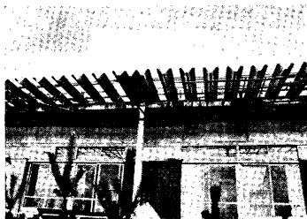
Photo. 11. Damage to roof: steel frame.
