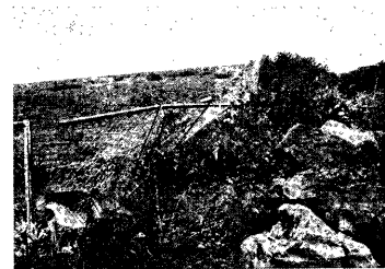
Photo. 16. Failure of net fence.
