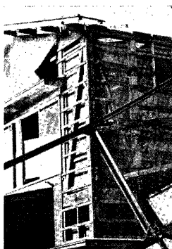
Photo. 3. Damage to external wall: wooden house.
