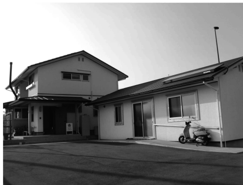
Fig. 1 Overall view of Kyo-Eco House with residential power system used for practical demonstration and analysis in this paper
