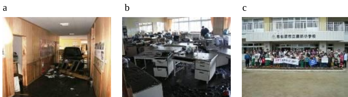
Fig. 6.4 Damage of Shishiori Elementary School (a) Hallway in front of Principal Room, (b) Staff Room destroyed by Tsunami, (c) School Garden Recovery Project with Volunteers of Bank
