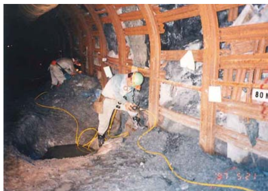
Photo 3 Installation of seismometers and cables near the fracture zone B in the survey tunnel excavated through the Mozumi-Sukenobe fault
