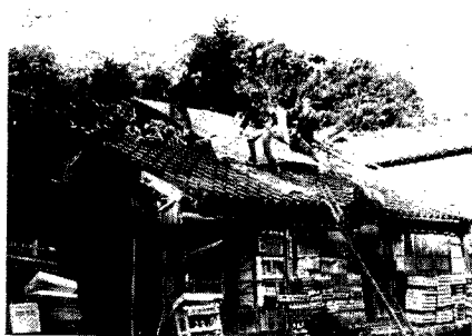
Photo. 4 Local damage to a wooden house.
