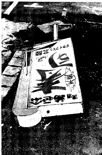
Photo. 6 Damage to the sign tower (1).
