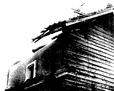
Photo. 2 Damage to a wooden house.
