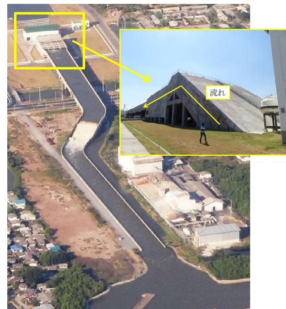
Fig. 3 Elevated canals near coastal area
