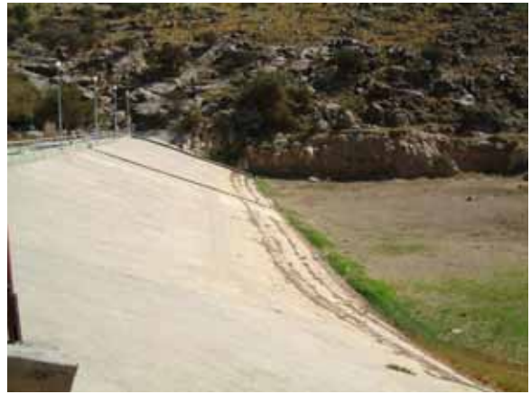
Photo 5 A facing type of rockfill dam
