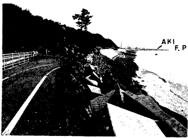
Photo.3 Breakdown of seawalls caused by Typhoons 7916 and 7920 at Aki Nishihama coast.
