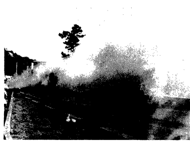
Photo.2 Wave overtopping by Typhoon 7920 at Nishihama coast.
