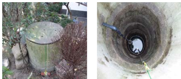
Photo 1 Digging type well
