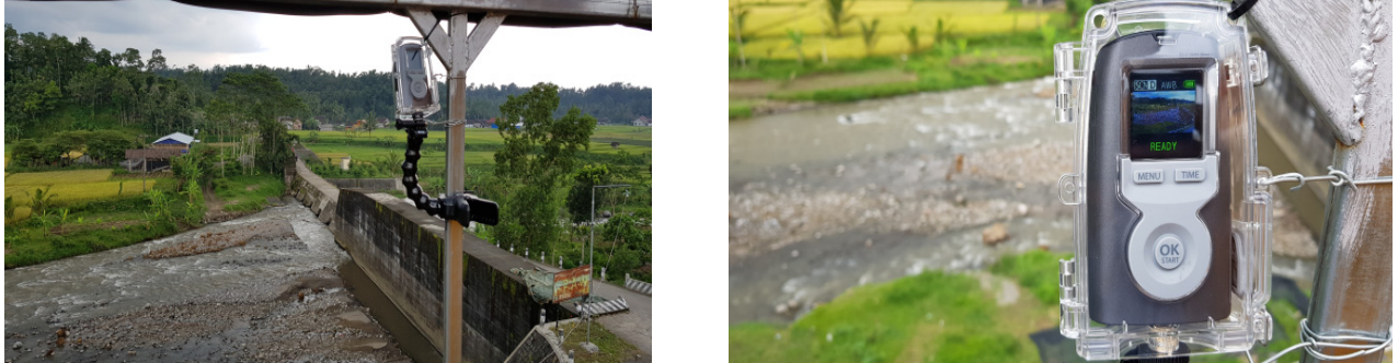
Figure 6. The installed monitoring camera at Lekso river
