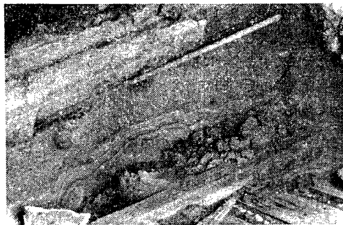
Photo. 7 Scene of the saw dust in layers in the ceiling.
