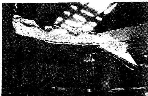
Photo. 6 Scene of accumulateing saw dust in the ceiling.
