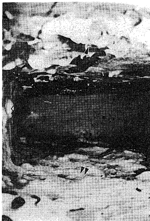
Photo. 2. Hyphal growth on the ground (⇐) and the supporting lumber (▶) for glass wool via a concrete foundation (⇐) under the floor.
