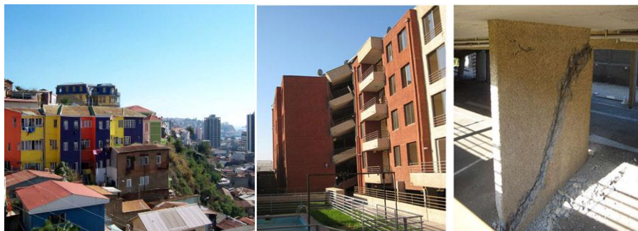
Figure 2.18 Adjacent buildings in a crowded city
