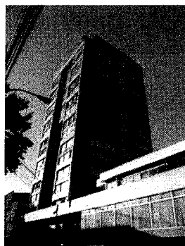
Photo 1 Appearance of Edificio Lincoyan
