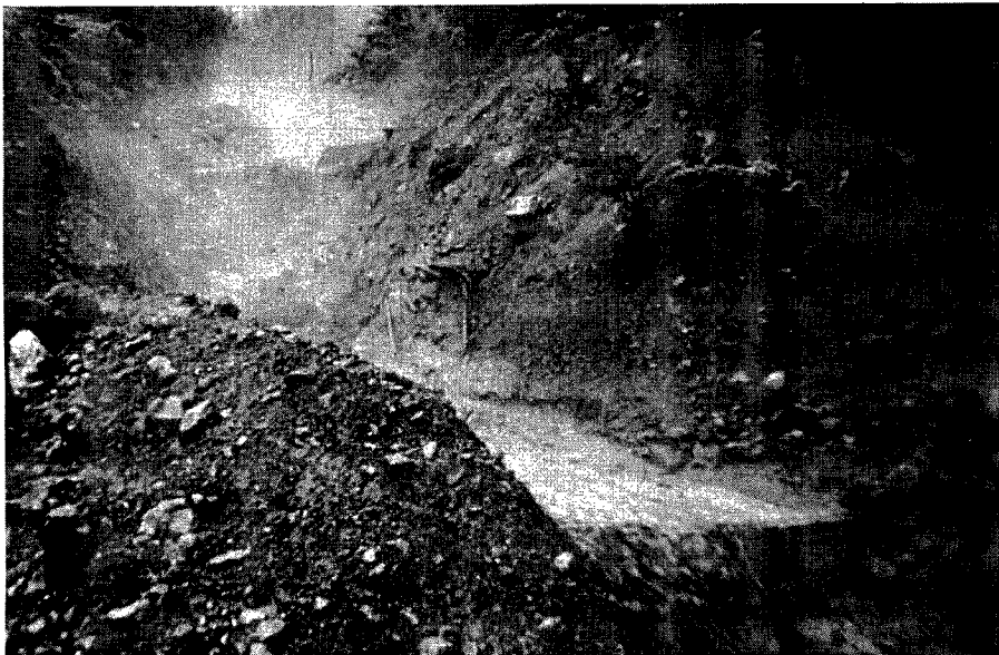
Photo. 8 Muddy stream flowing over dam No. 6 (lower dam) immediately after passing of mudflow front.
