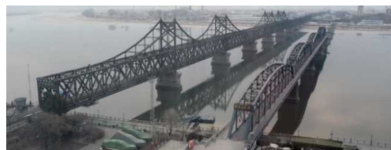
Fig.2 Present Yalu river bridge 1) .
