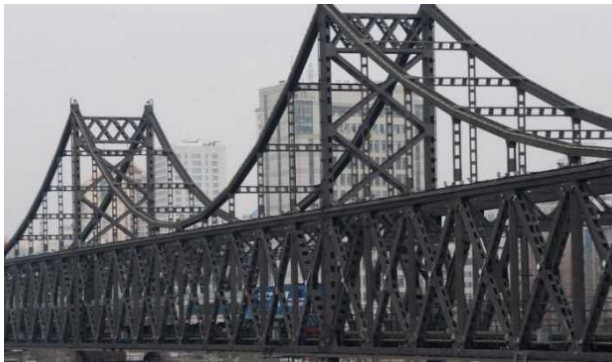
Fig.13 Bridge truss members and suspension structure of Yalu river bridge (Photo taken by Prof. Y. Takahashi)
