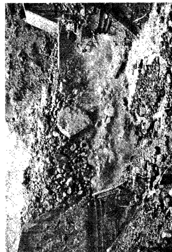
Photo. 3. Head part of debris flow running down over dam No. 6 upper (a series photograph taken every one second at 17h 34m, Aug. 3, 1976).
