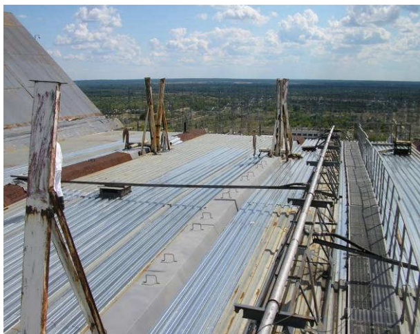
Fig. 10. Repair of the light roof (measure w/n)
