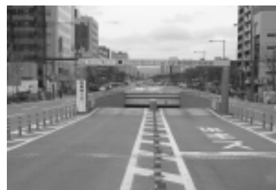
Fig.16 Entrance of underground parking lot
