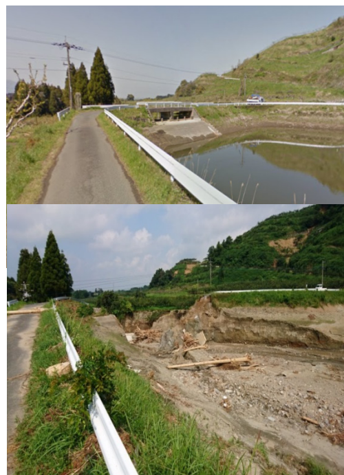
Photo 2 Collapsed Yamanokami irrigation pond (Naragatani River) (Upper : Before collapse (Google Earth) , Down : After collapse)
