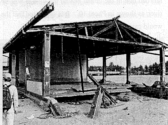
Photo 14 Damaged concrete floor by the tsunami lift force
