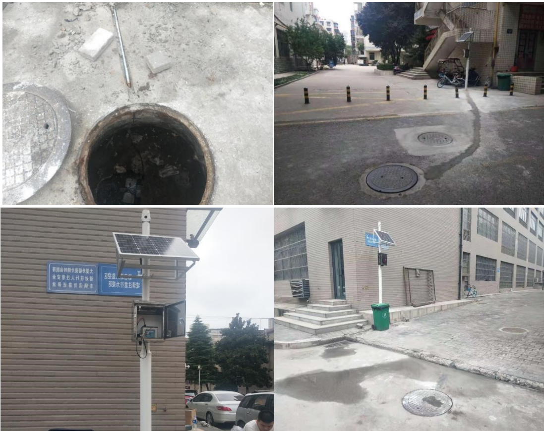
Figure 6 Construction process and effect
