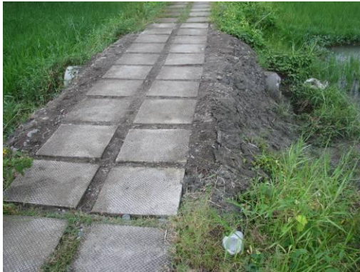
Fig. 3 The conditions after repair
