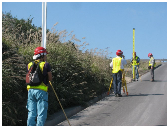
Photo 1 Basic members during leveling survey
