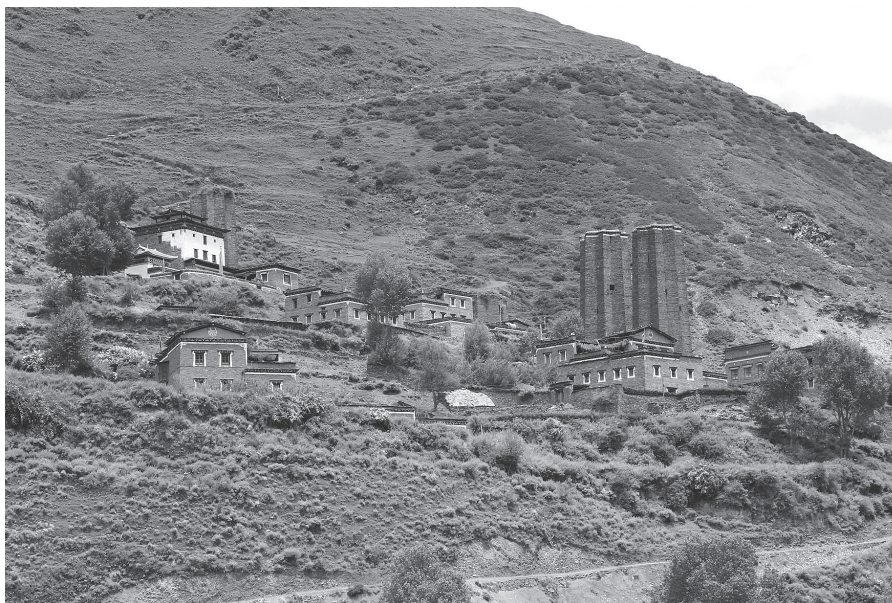
Stone towers near Pengbuxi village on the side of the Liqu river.
