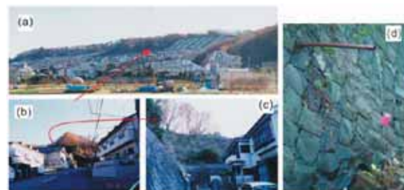
Fig.29 (a): a general view of the developed residential area. The red arrow indicates the location of the extrusive ridge, (b): front view of the ridge, (c): side view of the ridge, (d) : ground water indicating that a saturated zone exists below the ridge because bedding planes in the area are almost flat.
