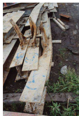
(c) Damaged H- steel for anchor head
