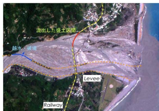
Photo 13 Situation after flooding and inundation
