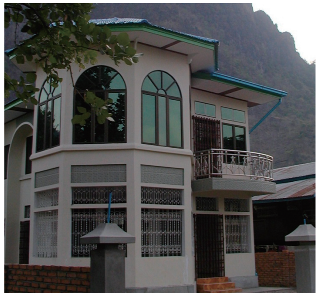
Fig. 2 A migrant-laborer’s house under construction
