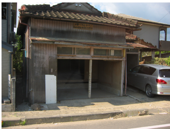
Fig. 6 Damaged house in the Torai area
