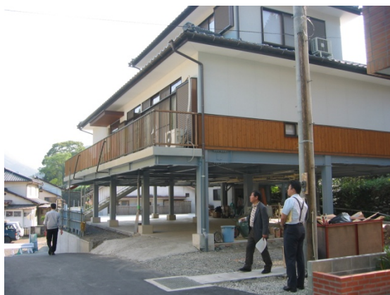
Fig. 9 A house that completed raising its floor
