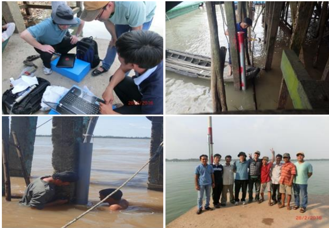
Figure 5.2 Field activities in installing additional turbidity and salinity stations. Photos were taken by Binh D.V. during the field trip in February 2016.
