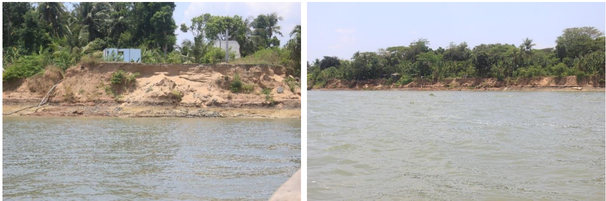
Figure 5.22 Typical severe river bank erosion in the VMD. Photos were taken by Binh D.V. during the field survey in April 2018.
