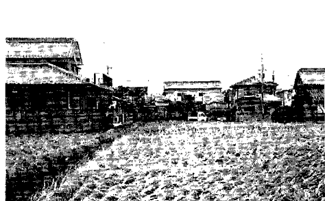
Photo 4 Fell down rice toward NE direction and damaged roofs of residential houses (Yamato-Takada city)
