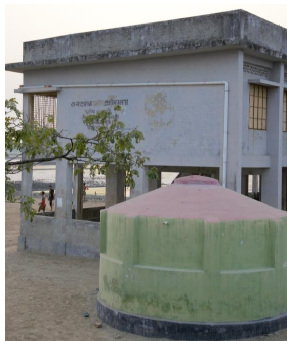
Photo 3 A rainwater harvesting system installed at a school
