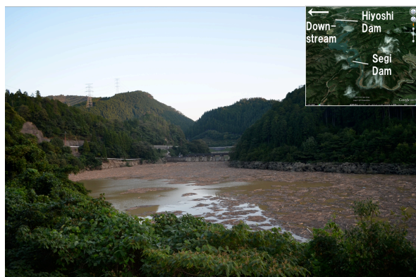
Photo 7 Accumulated driftwoods just downstream of Segi dam.
