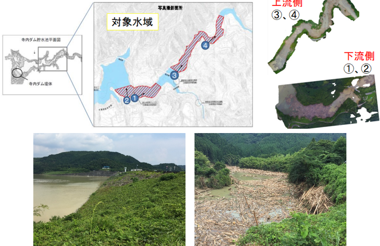
Fig. 1 Woody debris accumulation in the Terauchi Dam (upper: spatial distribution in the reservoir, lower left: downstream side of the reservoir, lower right: upstream side of the reservoir)
