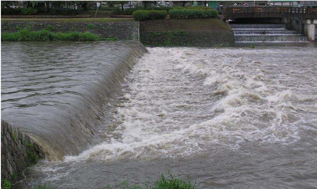
Figure 3.1 Abrupt expansion of flow downstream a step in the Kamo River.
