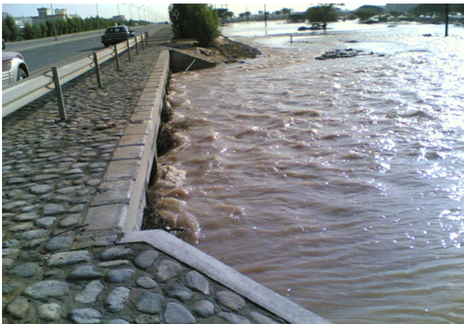
Figure 7.3 Flow through culverts during flood seasons.
