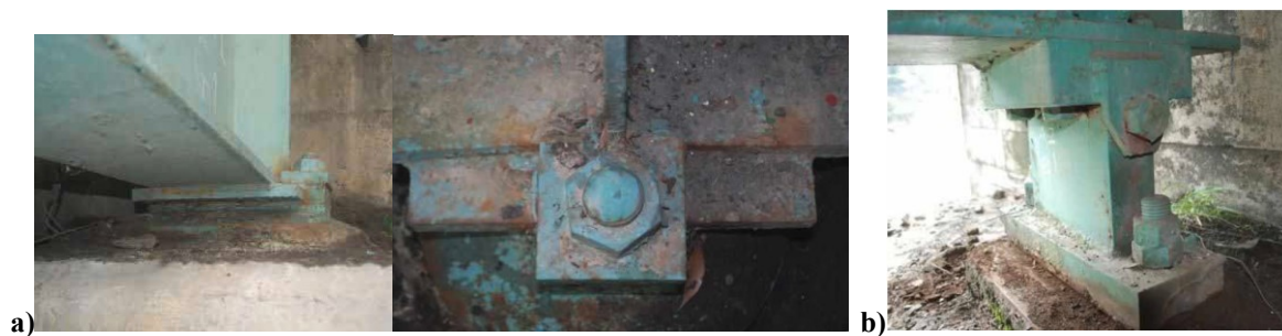
Figure 7.2 Photographs of the supports: a) on Ab1 abutment; b) on Ab2 abutment.
