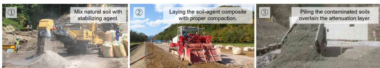
Figure 2.5: Representation of the construction process of the attenuation layer. Photo retrieved Feb 1, 2020, from https://cpds.kentsu.co.jp/technology/detail?id=40
